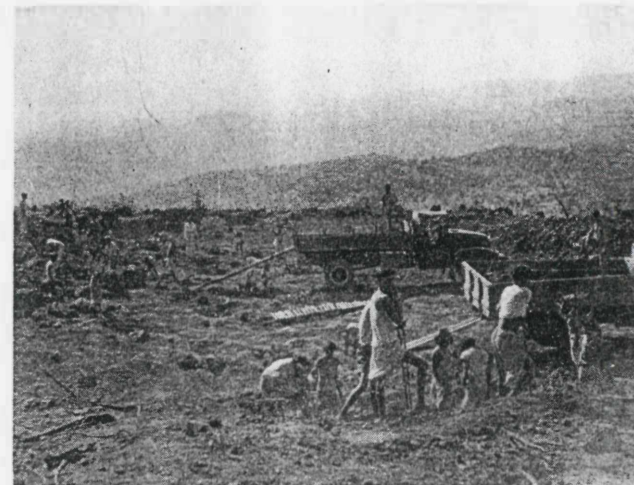
Removal of overburden in progress
